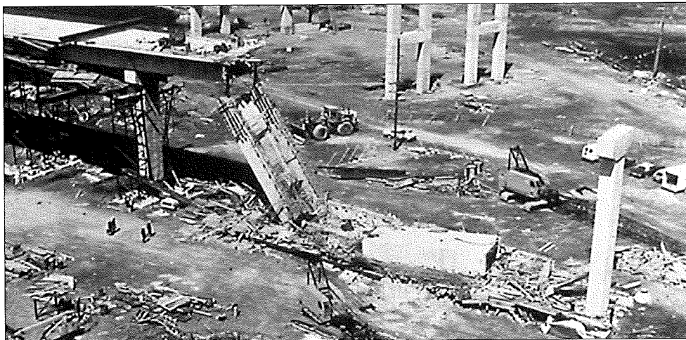
Fotografía 12. 912 Interstate Bridge Indiana Photograph 12. Bridge on I-912 in Indiana, USA
