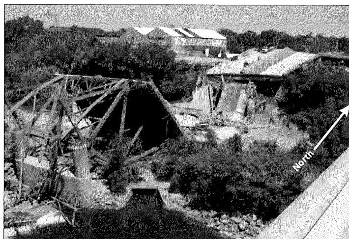
Fotografías 37, 38 y 39. Puente de Minneapolis (EE.UU). Vistas del puente colapsado Photographs 37, 38 and 39. Bridge on I-35W at Minneapolis, USA, after collapse
