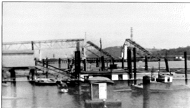
Photograph 8. Second Narrows Bridge, Vancouver, Canada Fotografía 8. Puente Second Narrows (Vancouver, Canada)
