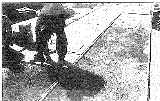
Figura 13. Enlosado Figure 13. Paver laying
