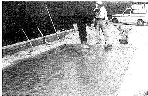
Figure 14. Grouting Figura 14. Enlechado
