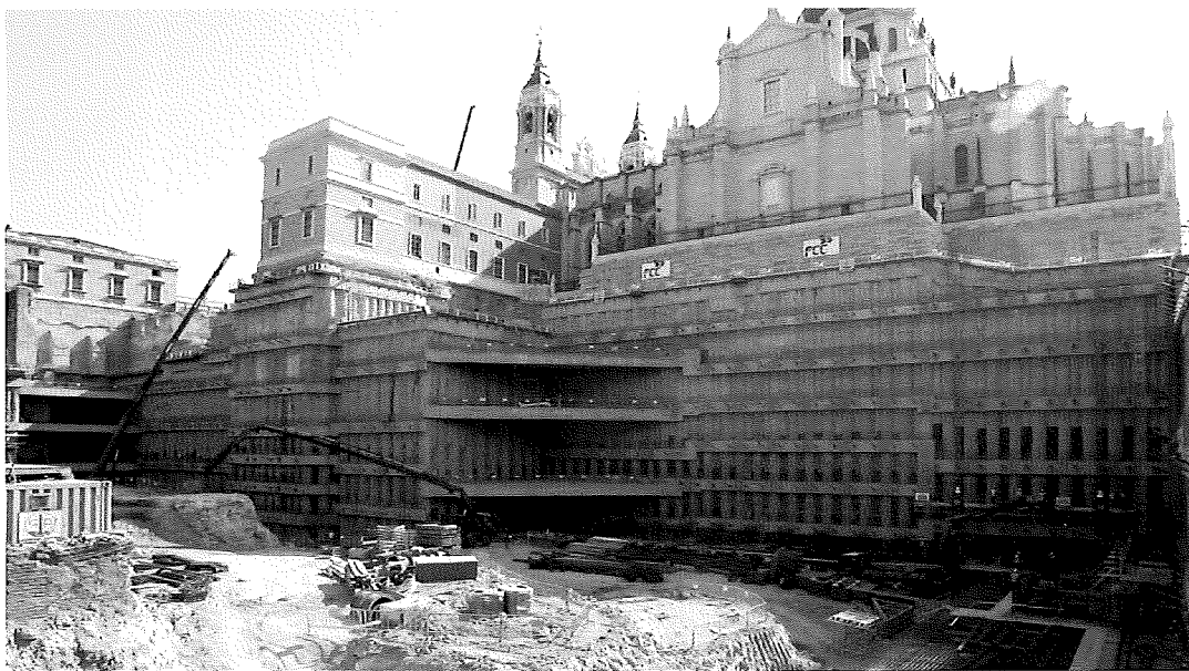
Figura 16. Vista general de codales Figure 16. Overview of angle braces
