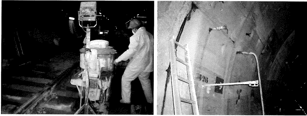
Photos 3 and 4. A posteriori injected waterproofing in a segment-lined tunnel
