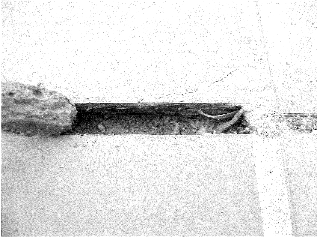
Figure 10. Faulty expansion joint (non-continuous cut, made through flooring only).
