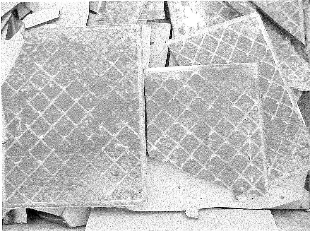
Figure 9. Back of the tiles in Figure 8, after removal.
