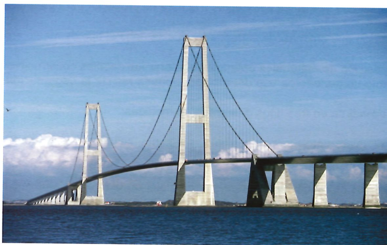
Figure 3: The Great Belt Link, East Bridge. Denmark
