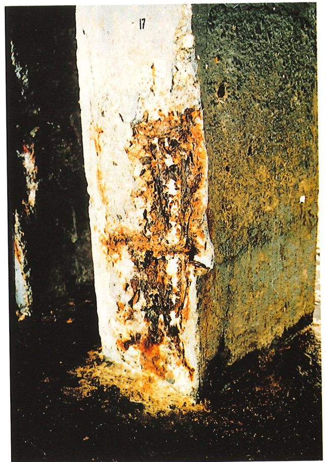
Photograph No. 8: Detail of a foundation pillar in a fish market, showing damage due to chemical degradation and reinforcement corrosion at the base only, caused by the pressure seawater used to clean the floor.
